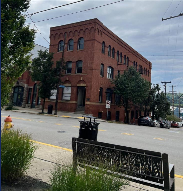
Lawrenceville office (3rd floor)
